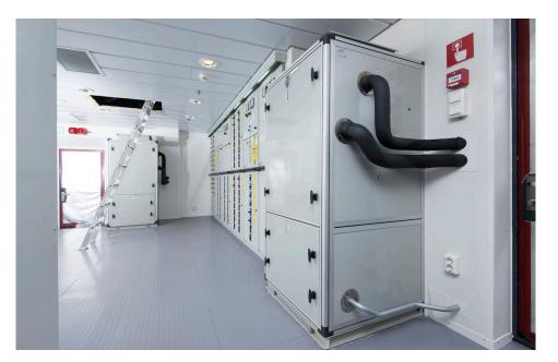
The COPRA Centrifugal fan coil (CFC) is constructed from painted double galvanized steel. It features a direct drive fan, Al/Al coil, high quality air filter on the inlet and an condensation drip tray.
