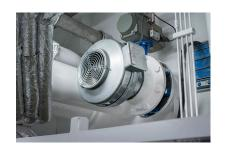
The straight through radial exhaust fan is compact and very easy to install. It can cope with high pressure and long duct runs, whilst still operating at low noise levels.
