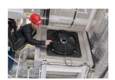
Axial Fan Coils are typically used in the Maritime Industry, specifically in technical spaces which have higher heating and cooling requirements.
